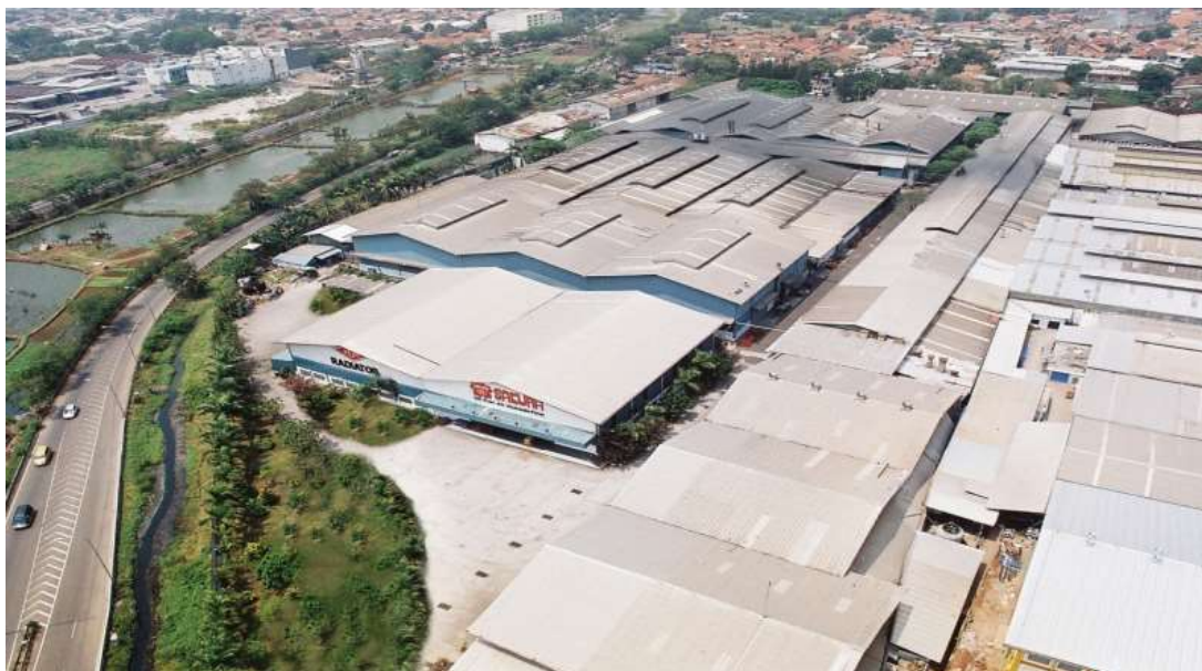
Kapuk Plant (Radiator Facilities)
